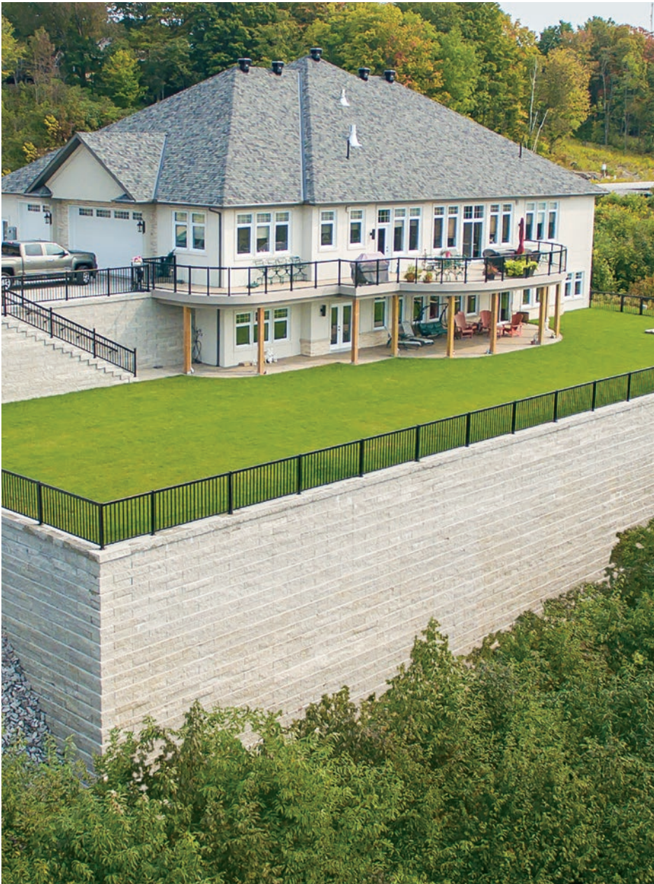
Split Coping and Wall (Coping overhangs one side)
